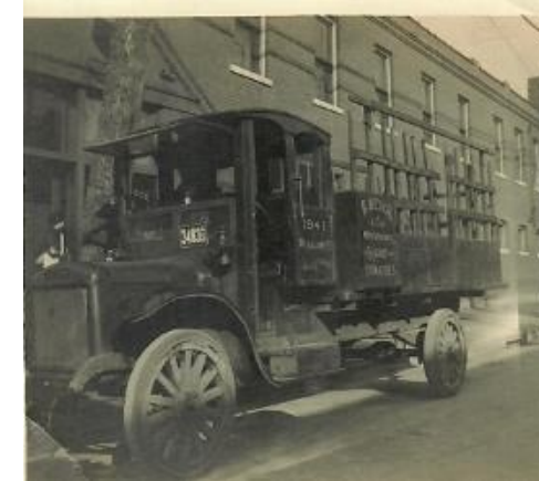
A. Weber & Company with Delivery Truck
